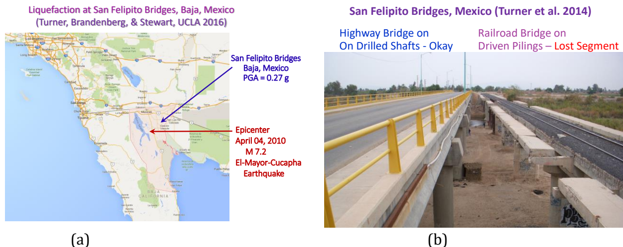
Figure 9.25: Liquefaction case study of Felipito Bridges, Mexico: (a) EQ epicenter and site location; (b) highway and railroad bridges (Turner et al. 2014)
